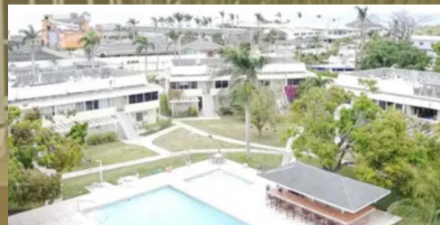
Seawind, Montego bay 1 units, one bedroom
